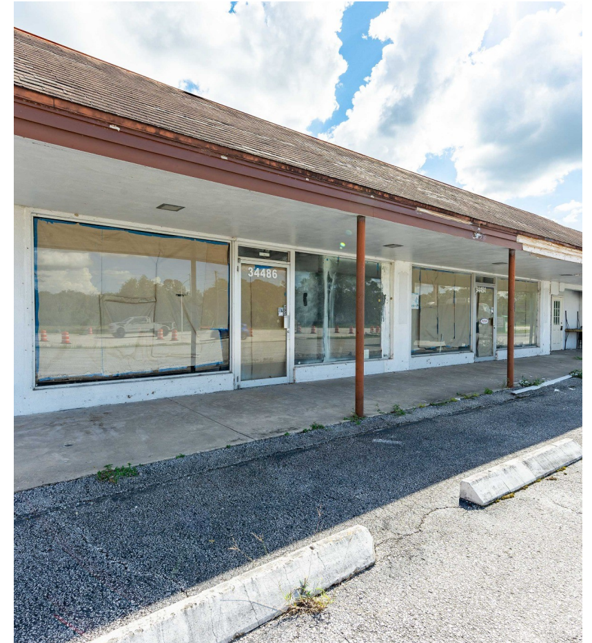
Close view of 34480 frontage
